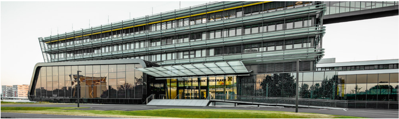
Raiffeisen multi function building, Raaba, built with ISOLAR NEUTRALUX® advance // Photo: © Arnold Glas
